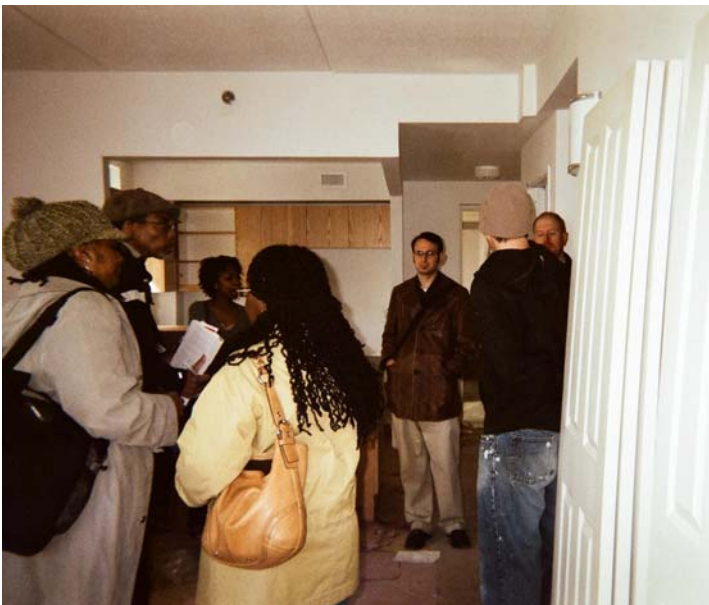
The Housing & Neighborhood Revitalization Committee checks out an apartment under construction
