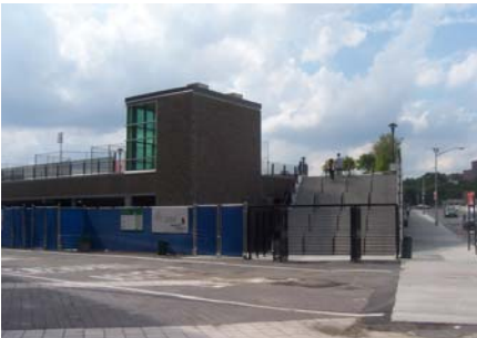
(Top) Rendering from Yankee Stadium final environmental impact statement showing stairs to a rooftop park above a parking garage. (Bottom) Project as being constructed now without even any viable space left for the landscaped screening shown in the rendering.
